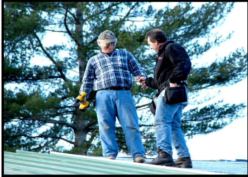
Noble Artie Dunham, our roofing contractor, and helper making good progress on the new metal roof for the Bektash Shrine Center. The entire roof is being replaced
